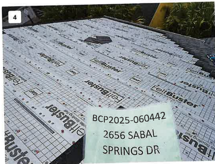
Project: 2656 Sabal Springs Dr Date: Jun 19, 2025, 4:36 PM Creator: Lucio Roofer
